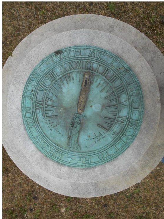
Moffat Sundial on top of monument with missing dial (2021)
